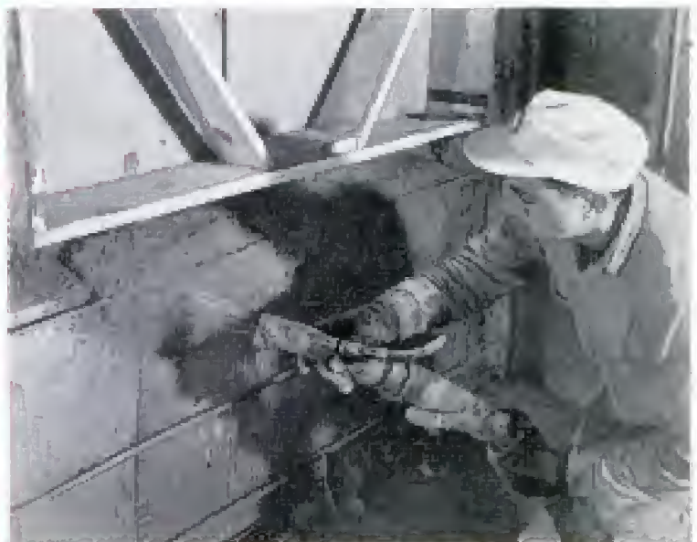
Perlite core fill for concrete blocks can double insulating effect of wall. Perlite insulation can't rot, decay or settle. Spraying machine below does the work of four plasterers. Light weight of plaster made with perlite makes spraying possible
